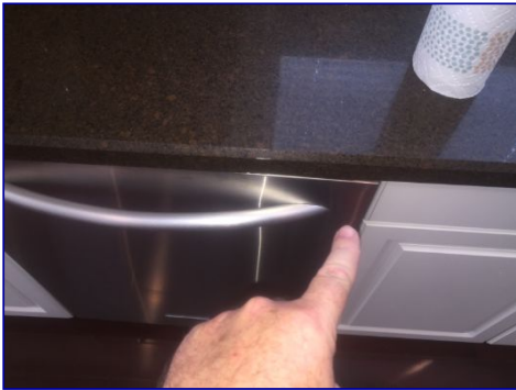
The dishwasher was not positioned properly. One side sticks out.
