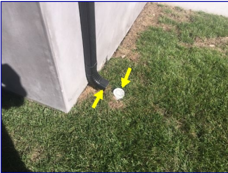
The rain gutter down spouts do not line up with the ground drains.
