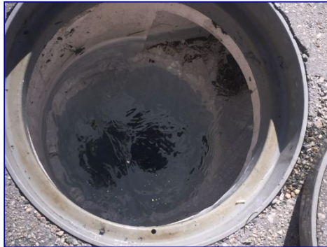
The pool water skimmer is missing a debris basket.
