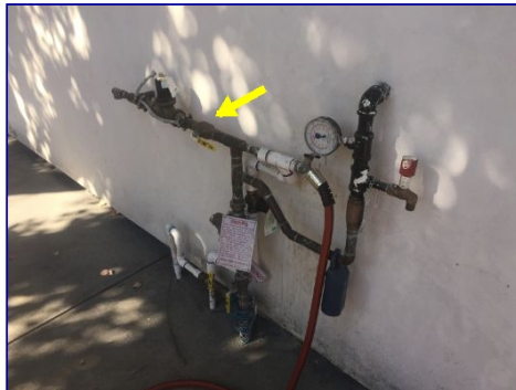
The home's fresh water shutoff valve.
