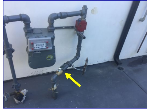
Gas line to backyard and pool heater.
