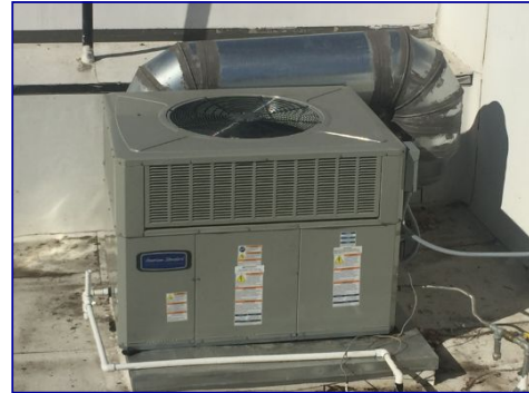
The home's North side furnace is an all in one and is on the roof.
