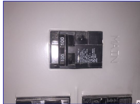
The sub panel in the laundry room is 100 AMP.
