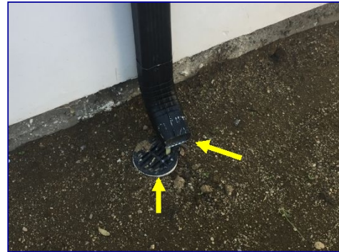
The exterior rain gutter down spout are not lined up with the ground drains.
