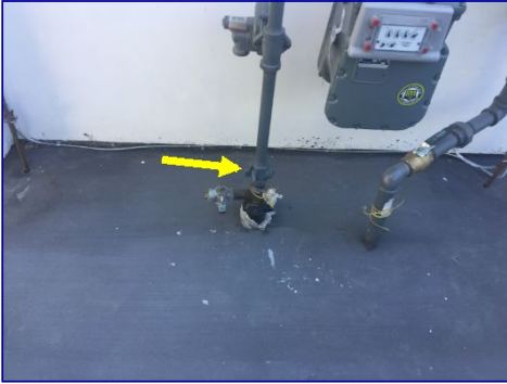
The natural gas utility meter and shutoff valve.
