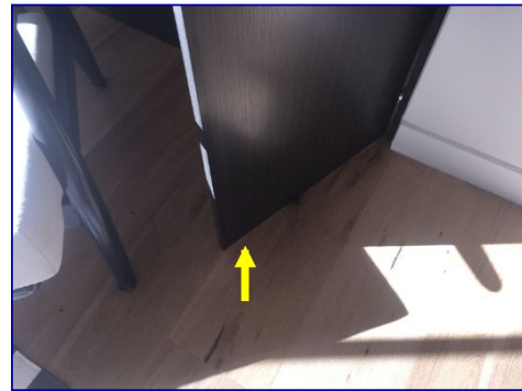
The Southwest bedroom closet door is too low to the ground and rubs the floor.
